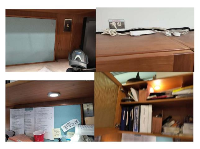
There is a small (approx. ¾") channel at the top rear of the cabinets to route the low voltage LED wires.
