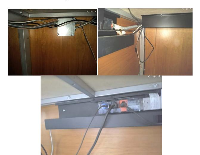
Computers are seated on the floor, with the keyboard, mouse, video wires, and computer monitor power are routed to the top of the countertop by access holes in the corners drilled into the countertop.
