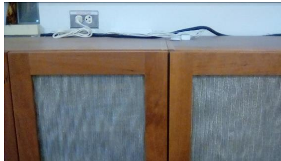
Power outlet above staff cubicle cabinet
